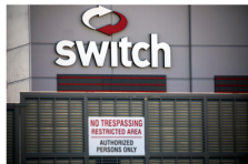
A Switch data center in Las Vegas on Nov. 7, 2017. (Jeff Scheid/The Nevada Independent)
