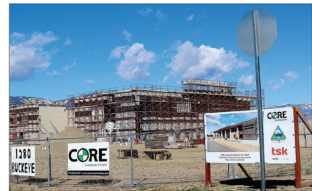
The Douglas County Justice Center rises along Buckeye Lane on Monday morning.
